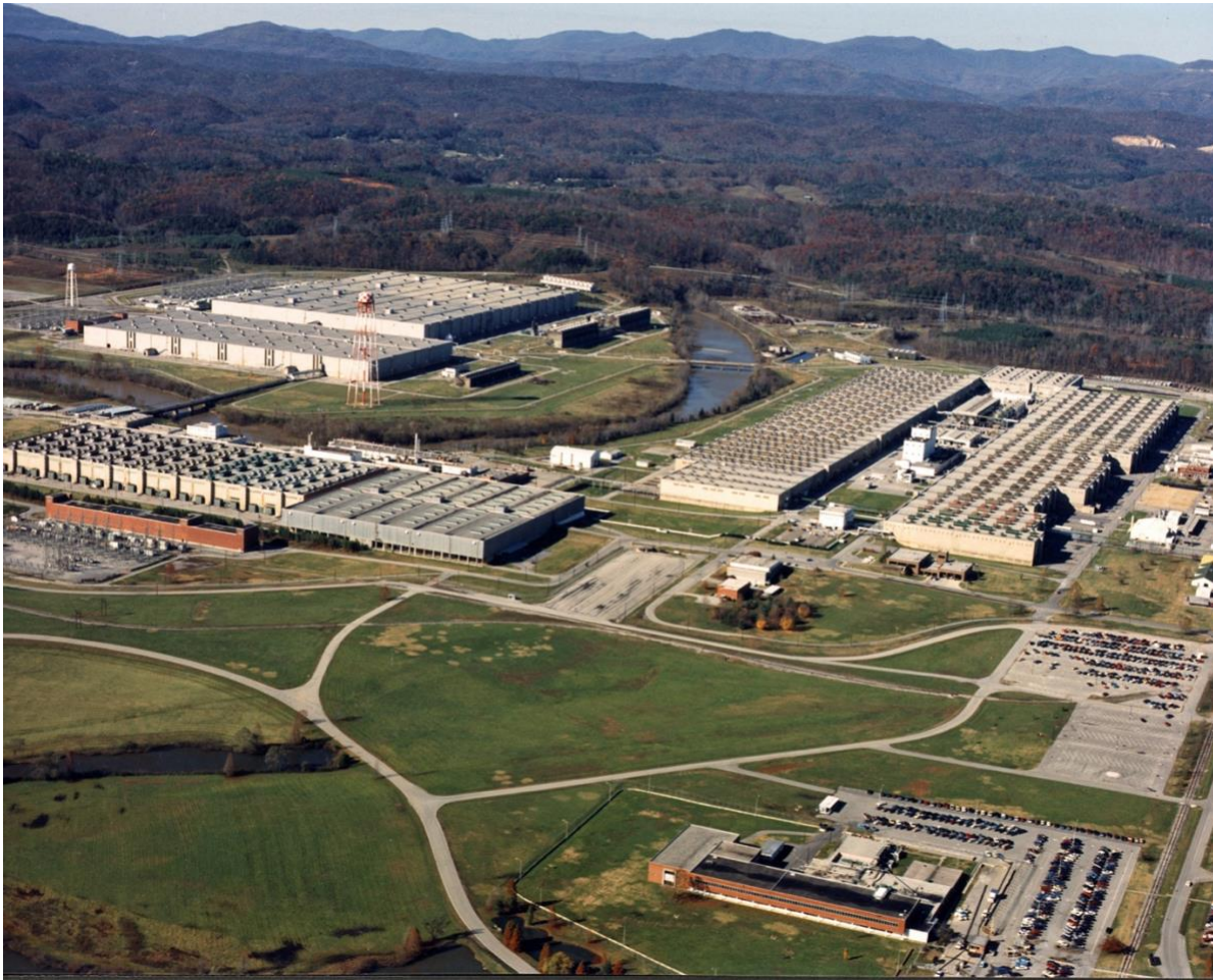
K-25 Gaseous Diffusion Plant including K-25, K-27, K-29, K-31, and K-33 gaseous diffusion process buildings (Photo courtesy of DOE)
